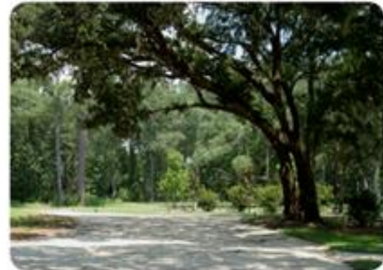
This Light Imprint parking lot provides a low tech solution using pervious stone. It is beautiful with or without vehicles.
