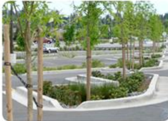
This conventionally engineered suburban parking lot has excessive grill costly infrastructure to support its rain gardens.
