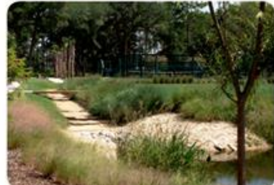
This vegetative and stone swale leading to a filtration pond is both a beautiful and more economical method of channeling and filtering stormwater. Light Imprint holes are generally categorised as intrinsically green holes.
